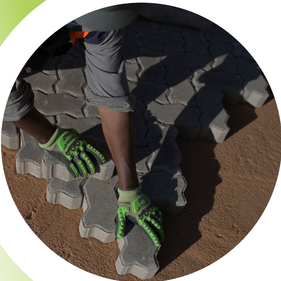
Pavement with blocks produced from Samarco tailings
